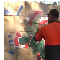
Graffiti is removed using just hot water at 2000 PSI / 2-3 gal per minute.
